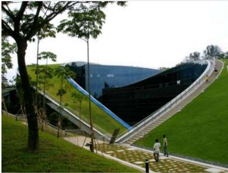
Fig. 3. Eco-school at Nanyang Technical University, Singapore
